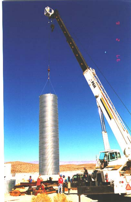
Mono-Pier Type Foundation
