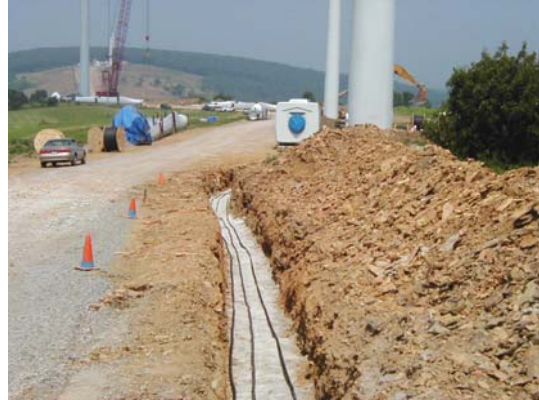
Typical Underground Cable Trench
