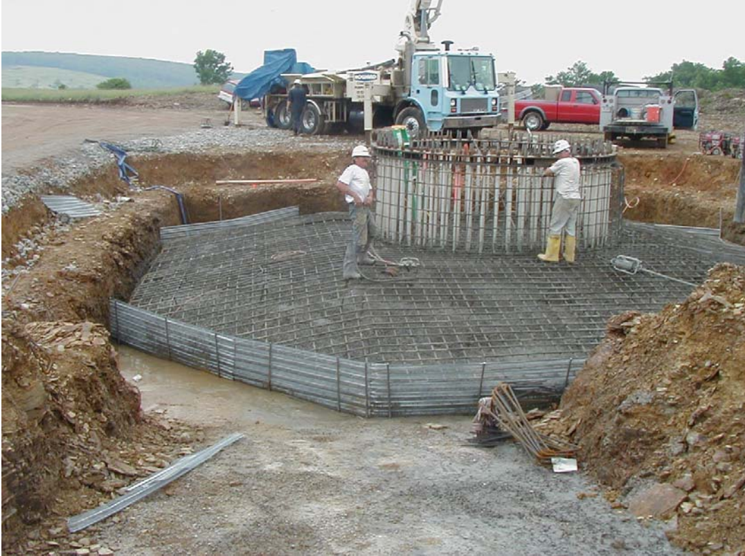
Spread Footing Type Foundation
