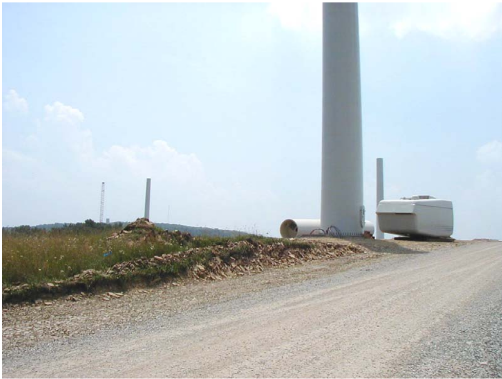
Typical Wind Power Facility Gravel Road
