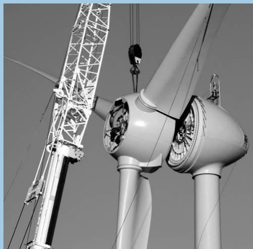
Wind turbine blade/rotor assembly lifted into position to be connected to the low-speed shaft.
